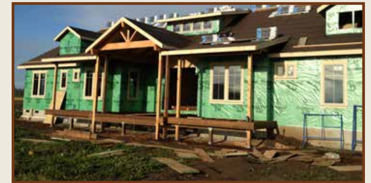
'Artistry' was built in about 6 1/2 months, including land infrastructure installation
