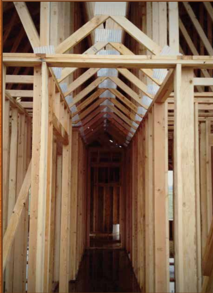
The vaulted hallway, pictured above, was built into the roof system.
