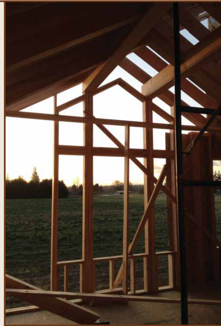
The Master Suite was timber framed to keep the roof pitch the same as the ceiling on the inside in order to match the angled tops of the windows.
