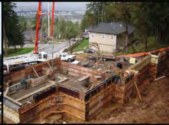
FOUNDATION ON FEB. 19, 2007
